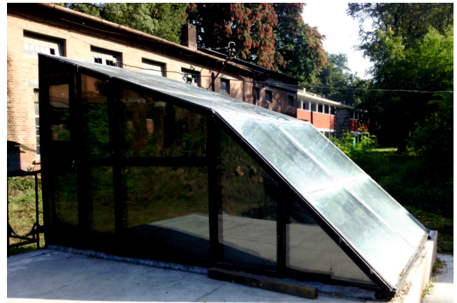
Figure 4: External view of the solar kiln showing double inclined roof (A), internal view of the kiln showing the aluminum fins attached to lower side of the roof solar collectors (B), G.I. sheet solar collectors fitted beside the kiln east/west walls (C)
