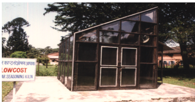
Figure 2: First commercial solar kiln developed by FRI in 1980
