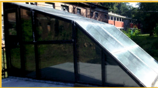
Head based storage Solar Kiln
