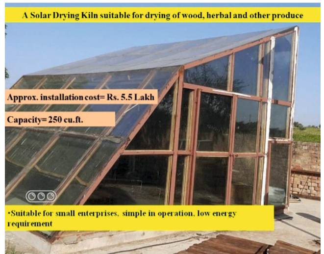
Fig. 6: The third generation kiln installed at Churu
