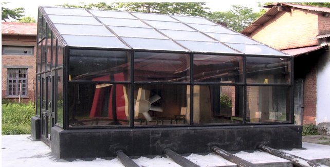
Figure 3: The modified single glass Solar Kiln for Timber Drying
